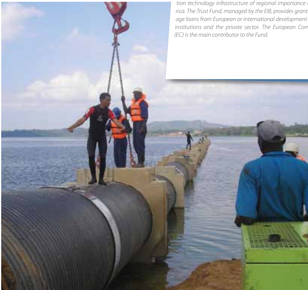
Gaba offshore pipeline, Kampala, Uganda
