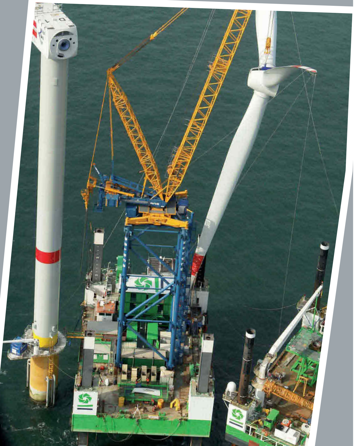
Offshore installation of a wind turbine, Belgium
